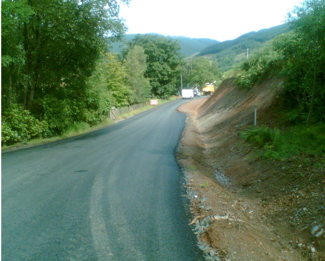
Artaraig area – Final surfacing works completed 1 st Aug
