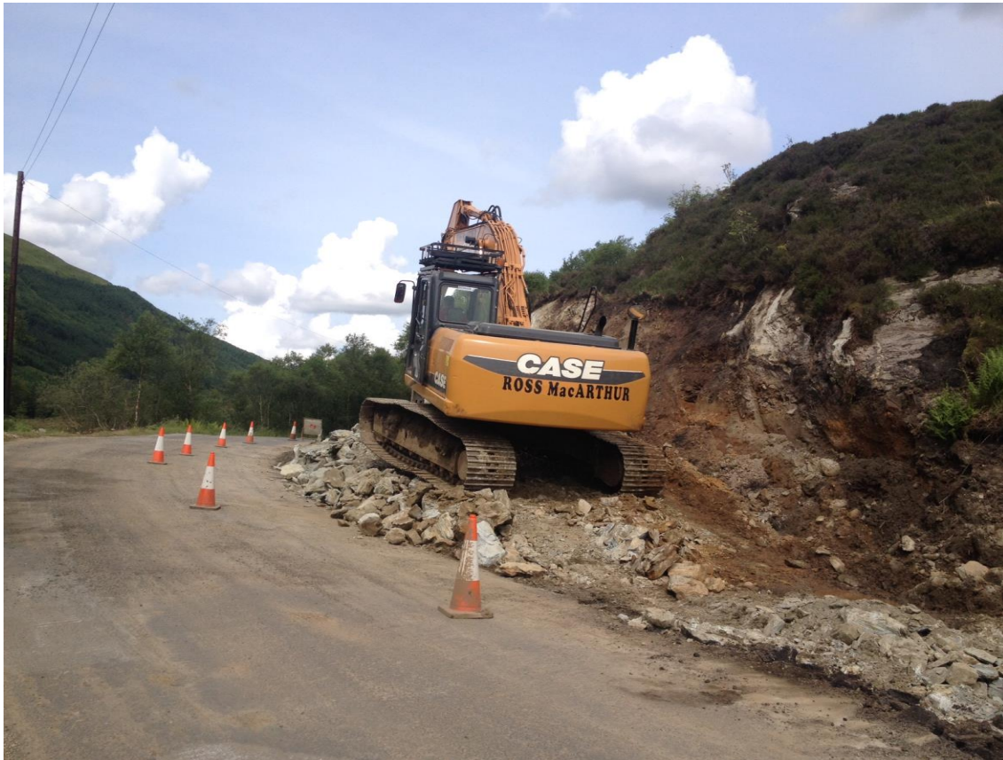
Rock excavation and C/W widening Clachaig – Glen Lean Flats 5 th June.
