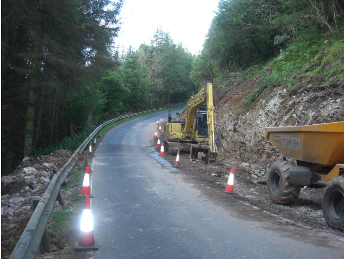
Earthworks and carriageway widening construction Craigendive Hill 27 th Aug
