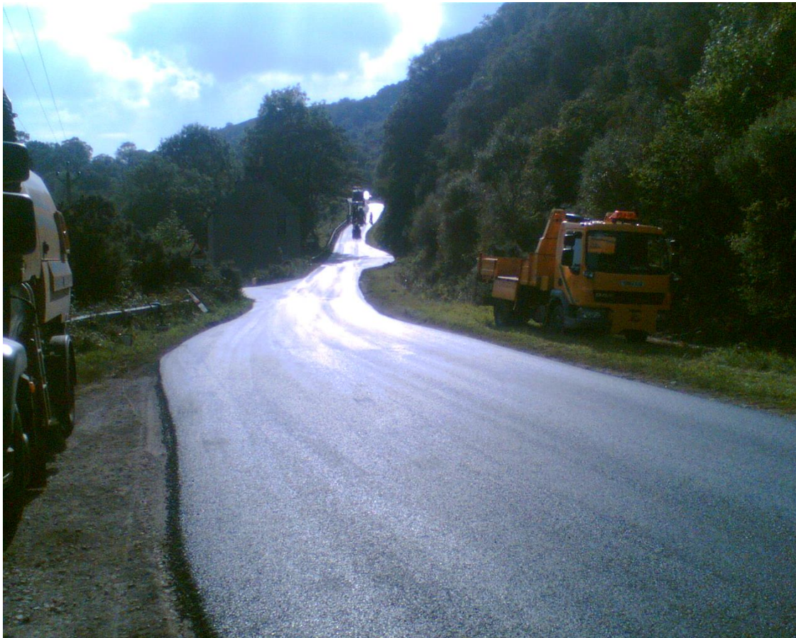
Foot of Craigendive Hill , final surfacing , 10 th September
