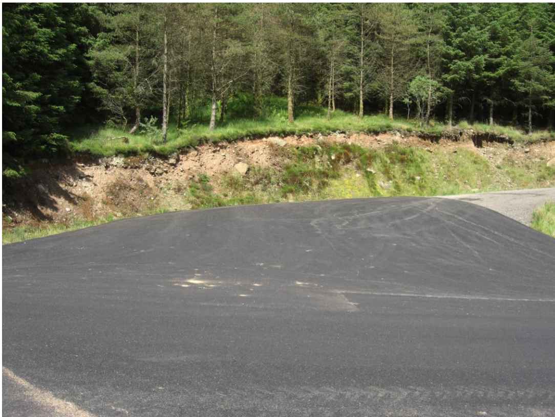
Glen Massan / Glen Tarsan Exit Point accommodation works , surfaced interface. 19 th June
