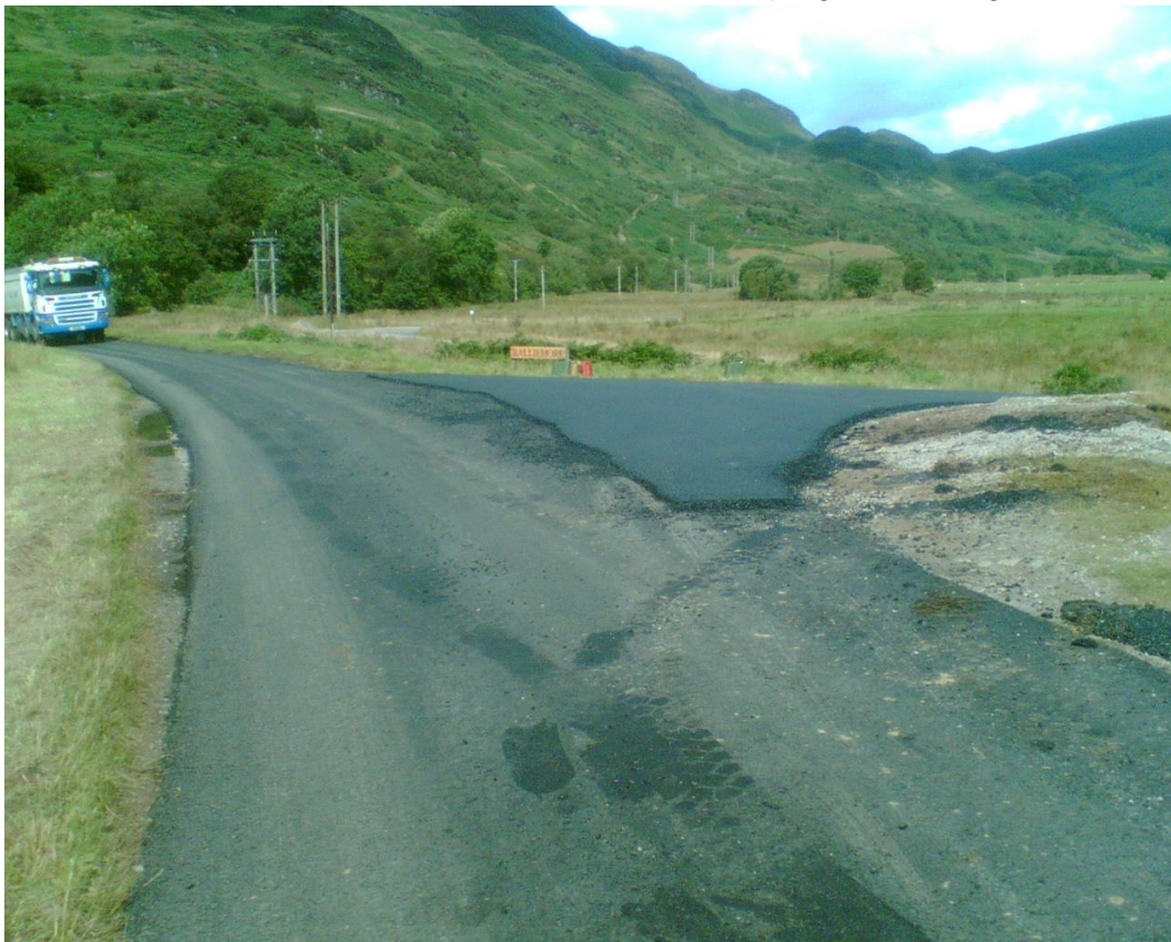
Balliemore Estate entrance accommodation works, in progress 1 st Aug
