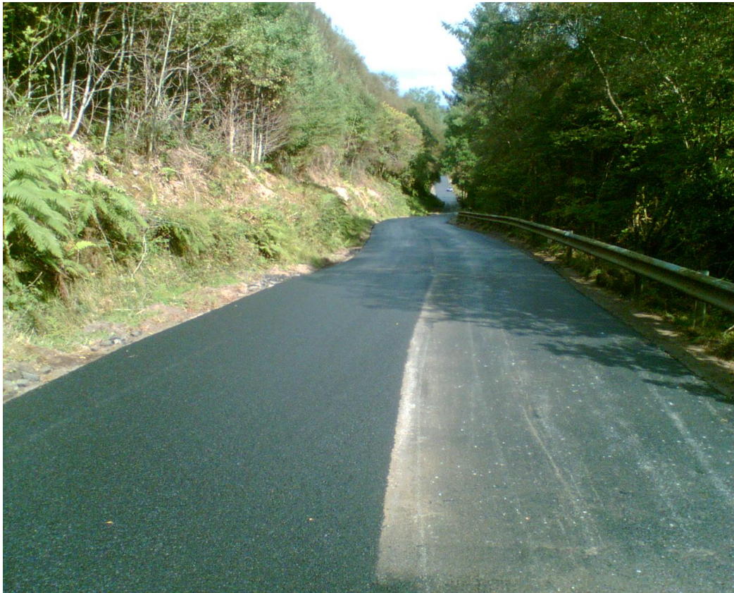
Central section Craighendive , widened to 2 lane 17 th September
