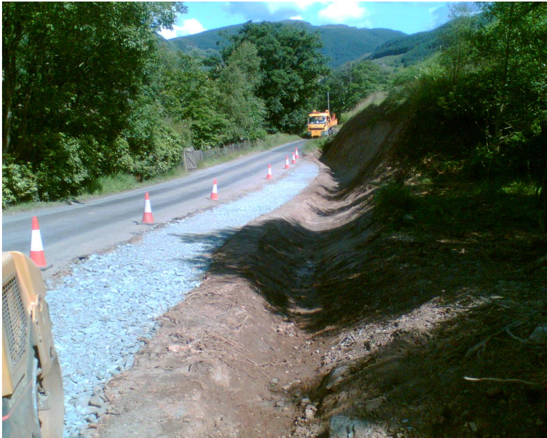
Glen Lean Flats – Balliemore - Ardtarig area , earthworks and widening 1 st July
