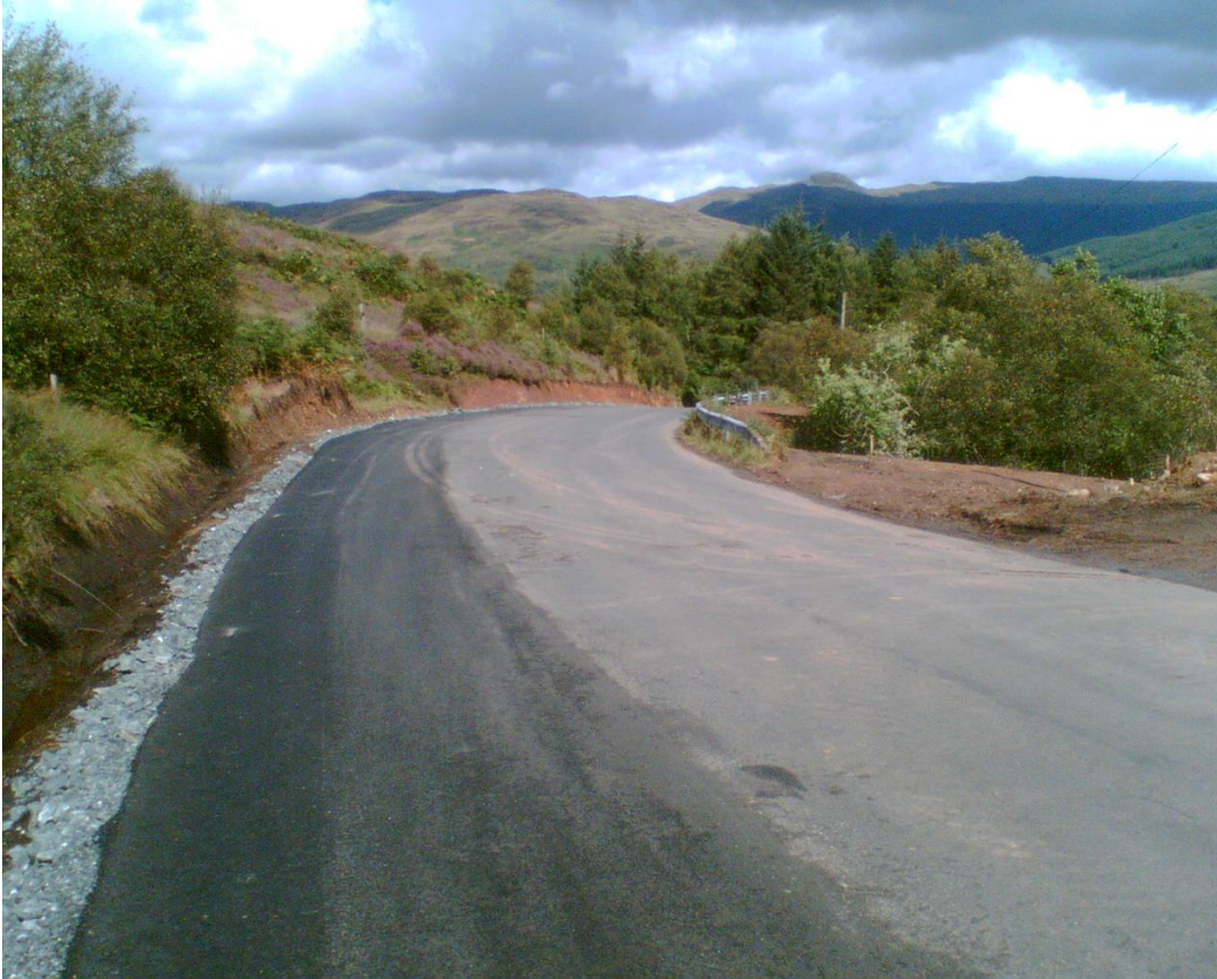
Widened section to 2 lane. Top of Craigendive Hill ( 18t Wt Limit ) 21 st August
